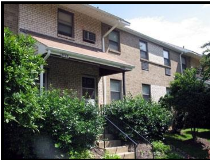
Exterior view of one of the 54 units at Emory Grove.
