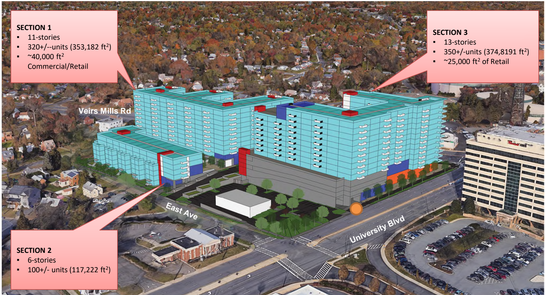
Aerial view illustrating the rear of the site that is comprised of Section 2 (foreground) along University of Blvd and East Ave.
